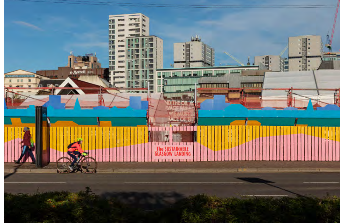
Site boundary: designed to attract the general public while providing a robust barrier to protesters and vehicle attacks.
